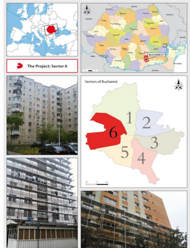
Project: BUCHAREST S6 THERMAL REHABILITATION - Romania
