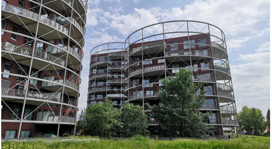
Picture: Conversion of an old gasworks into social housing, Hilversum Photo Credit: Housing Europe
