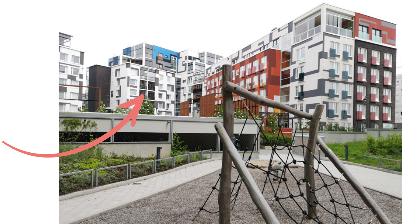
Picture: Communal playground and view of social housing – Jätkäsaari District (Helsinki) Photo Credit: Housing Europe
